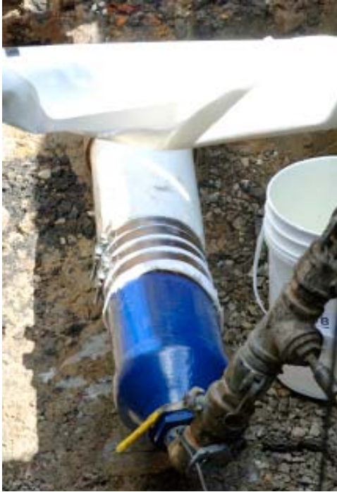
Elastollan ® ET 3685-11 - Hotmelt TPU adhesive for CIPP potable water rehabilitation application.
