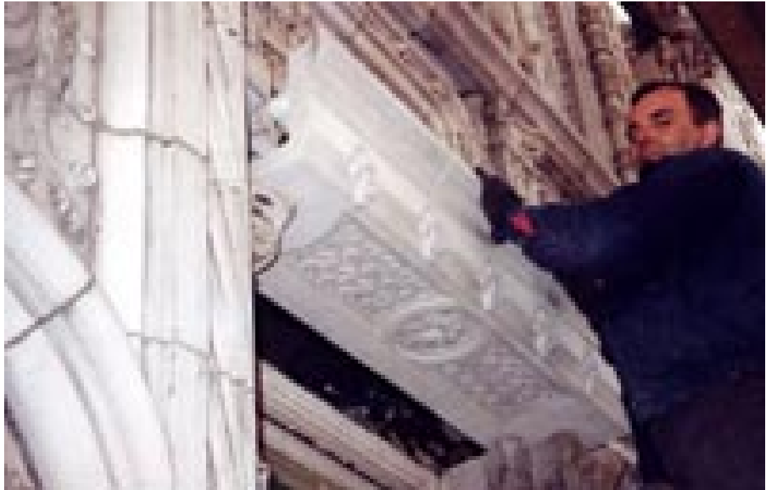
Using MetaMax in conjunction with other additives enables the concrete to have compressive strengths over 6,500 psi and only half the water absorption of ordinary concrete.
