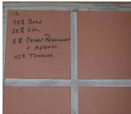
5% MetaMax ® EF @96 hours, Slight efflorescence
